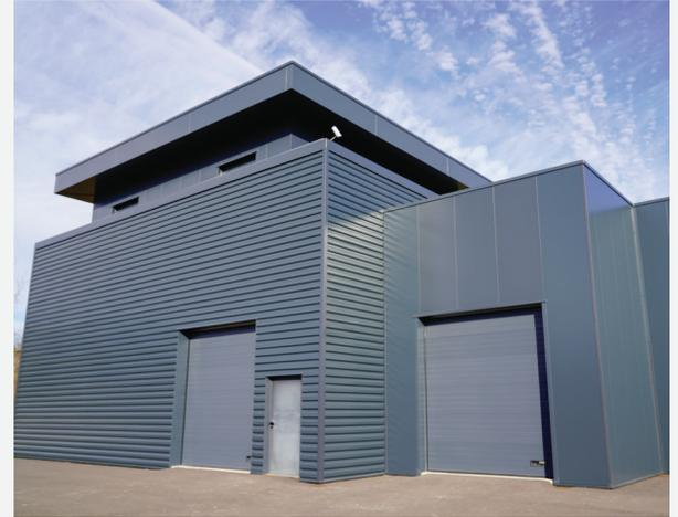
Elevation, Pinnacle, and Summit Series panels are interchangeable with the **Proprietary WaardLok Fastening System**. It is designed to guard against wind-driven rain and wind uplift.
